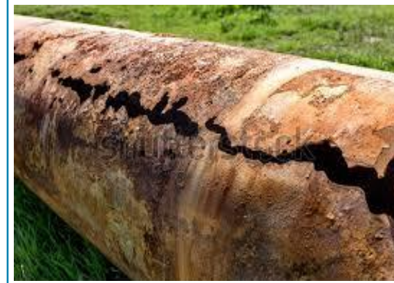
High operation and maintenance costs, disrepair and service failure
